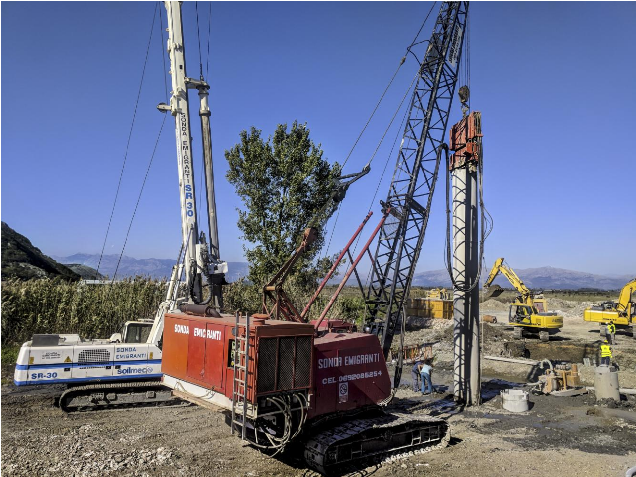
(Piles with bentonit and vibration casing in Velipoj-Shkoder)
