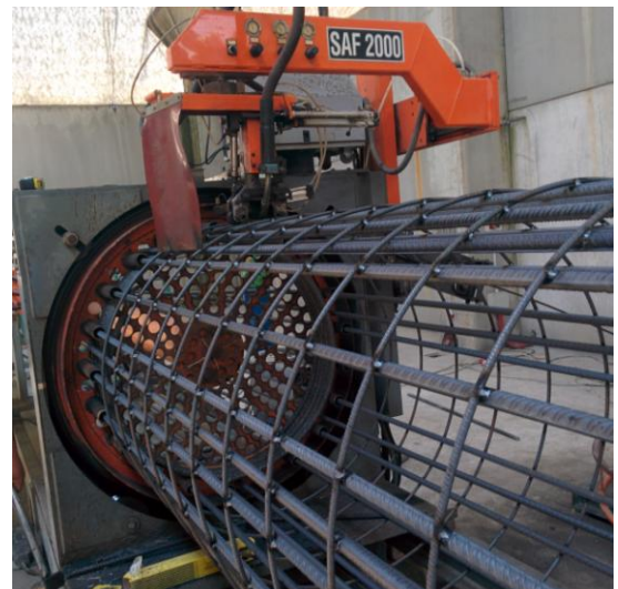
(welding the rebars on our site)
