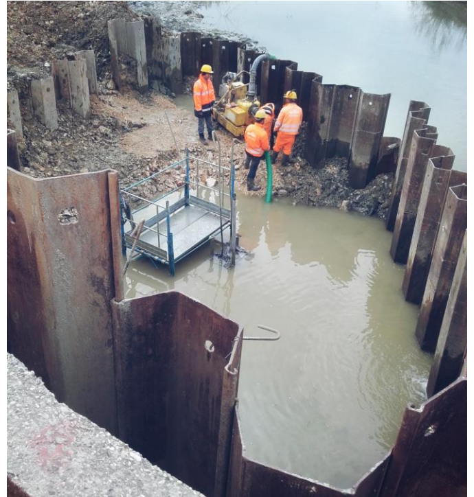
(protection of pier of bridge for TAP project in Seman, Fier.)
