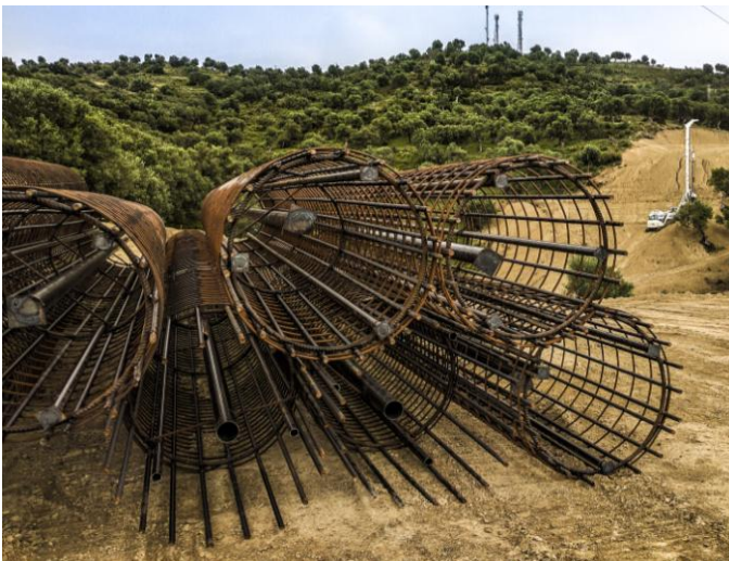
(cages with sonic test pipes, 1000mm)
