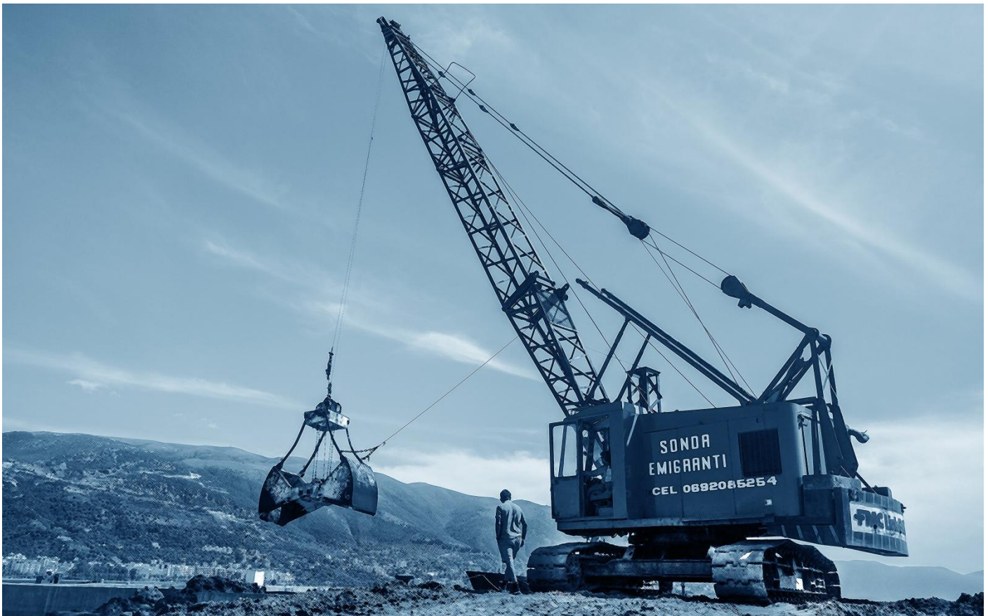
(Mr. Hoxhaj was chacking the Dredging in port of Vlora)
