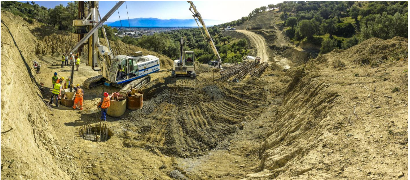
(Bridge on ByPass Vlore 1200 mm for 20 meters)
